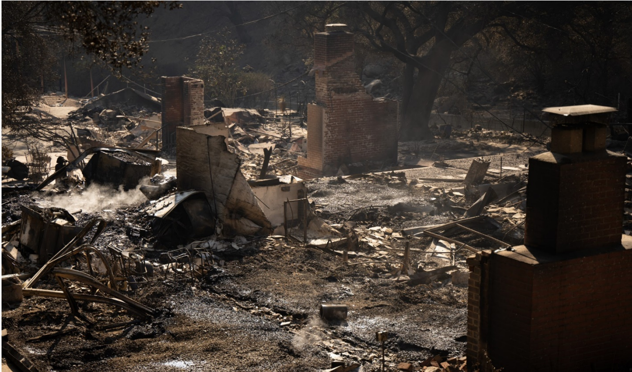
Damage from the Eaton Fire. US Air National Guard Photograph by Tech. Sgt. Joseph Pagan.
